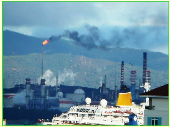
CEPSA Refinery flares in December 2009
